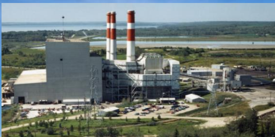
1956 – Commissioning of our first large, centralized coal-fired plants
