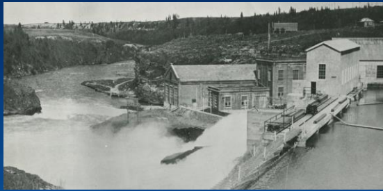
1911 – Construction Of Calgary Power's first hydro plant on the Bow River
