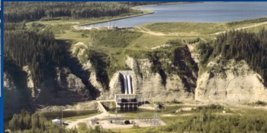
1965 – Brazeau Plant commissions first turbine
